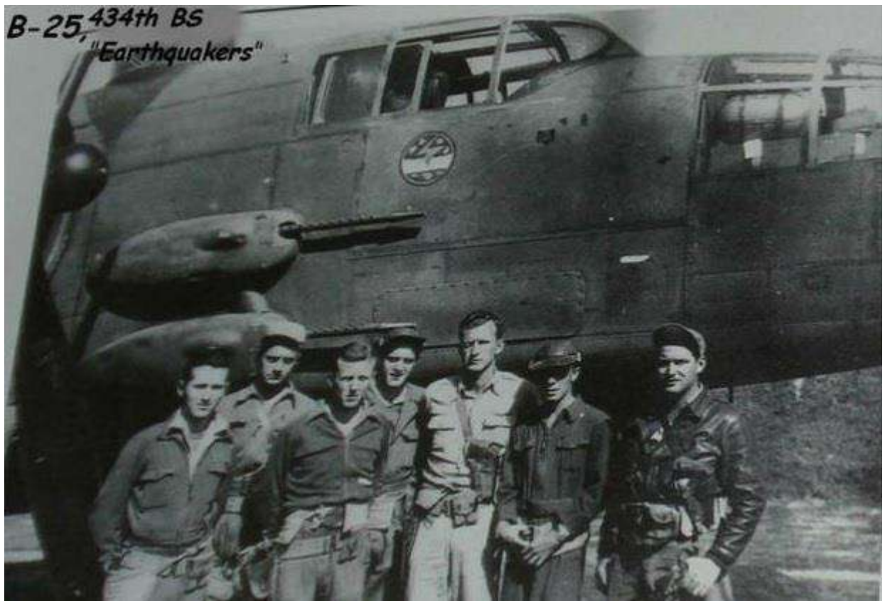
434th BS "Earthquakers"
